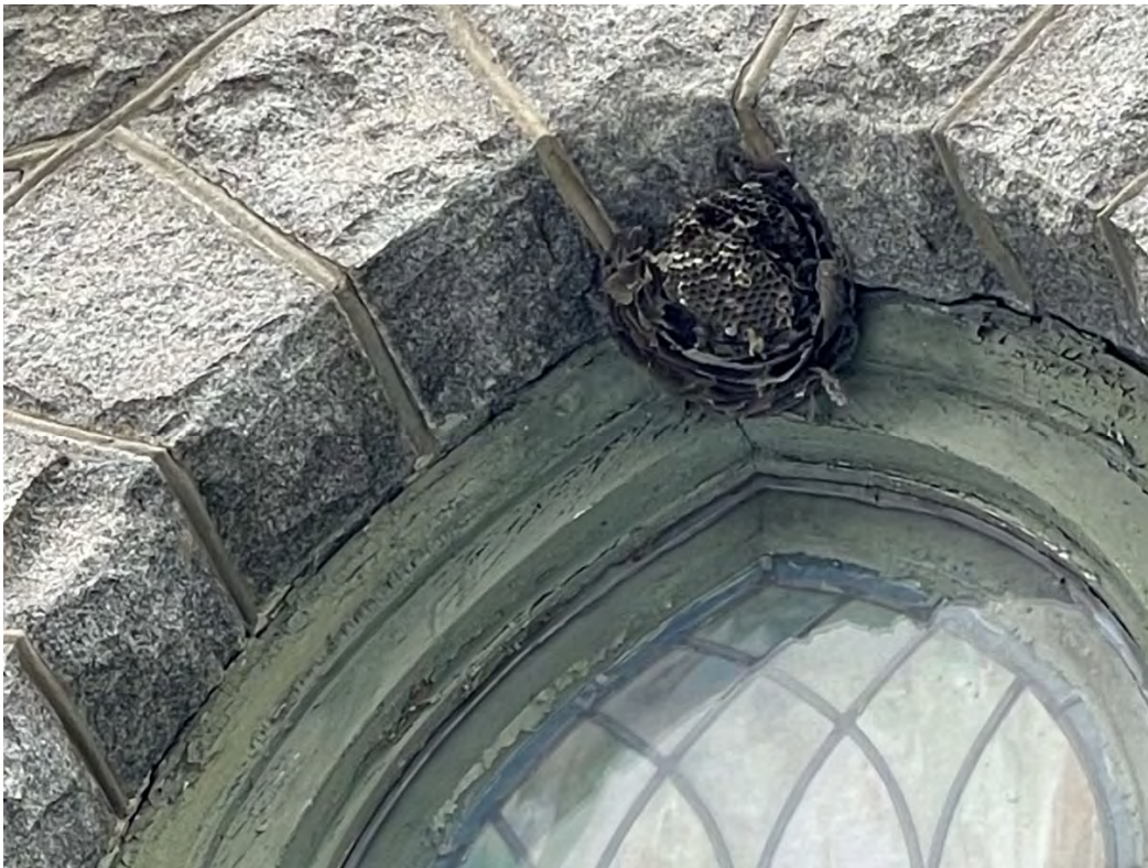
Granite Church – Existing Conditions – Doors and Windows First Floor - Double-Hung Stained-Glass Chancel Window - East-most Chancel Window on South Elevation Insect Nest; Acrylic Sheeting on Exterior of Window Could Cause Heat Build-up and Damage to Window
