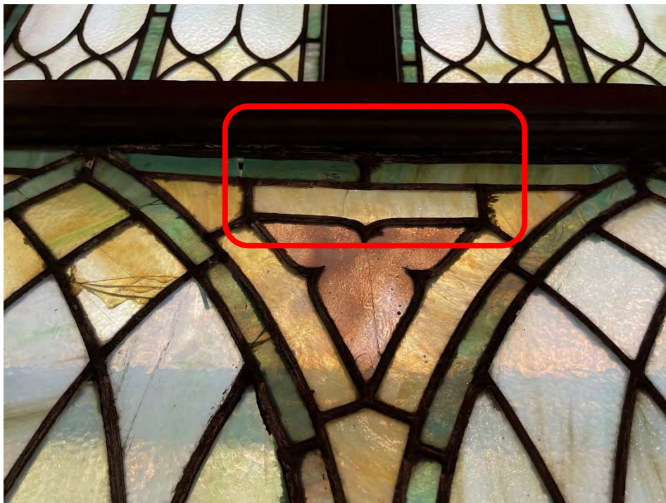
Granite Church – Existing Conditions – Doors and Windows First Floor – Double-Hung Stained-Glass Window on West Wall in Sanctuary – Window Second from South Separation of Window from Frame at top of Bottom Sash
