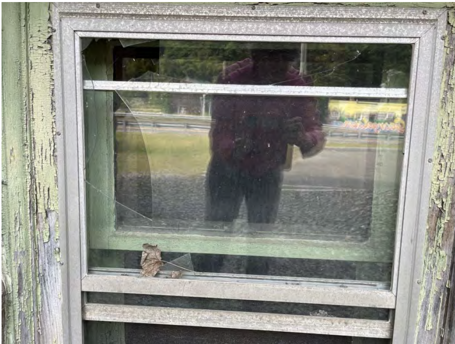
Granite Church – Existing Conditions – Doors and Windows Basement – Double-hung Window in Stair Hall Broken Glass in Storm Window – Wood Frame in Need of Painting
