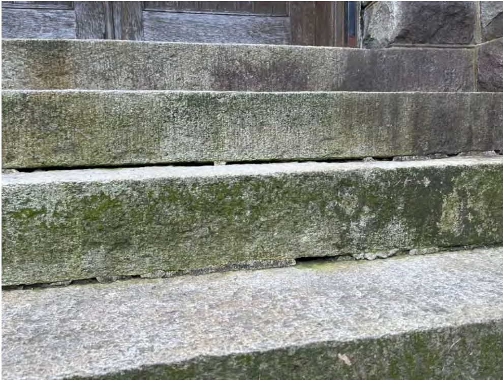
Granite Church – Existing Conditions – Exterior Masonry North, Main Entrance Steps – Open Joints in Steps
