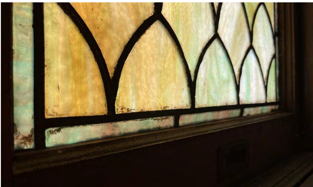
Granite Church – Existing Conditions – Doors and Windows Typical Double-Hung Stained-Glass Chancel Window First Floor - Deflection of Lead Comes and Glass at Base of Window
