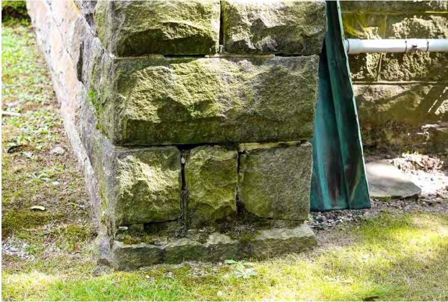
Granite Church – Existing Conditions – Exterior Masonry West Elevation – North Buttress – West Face - Open Joints and Staining
