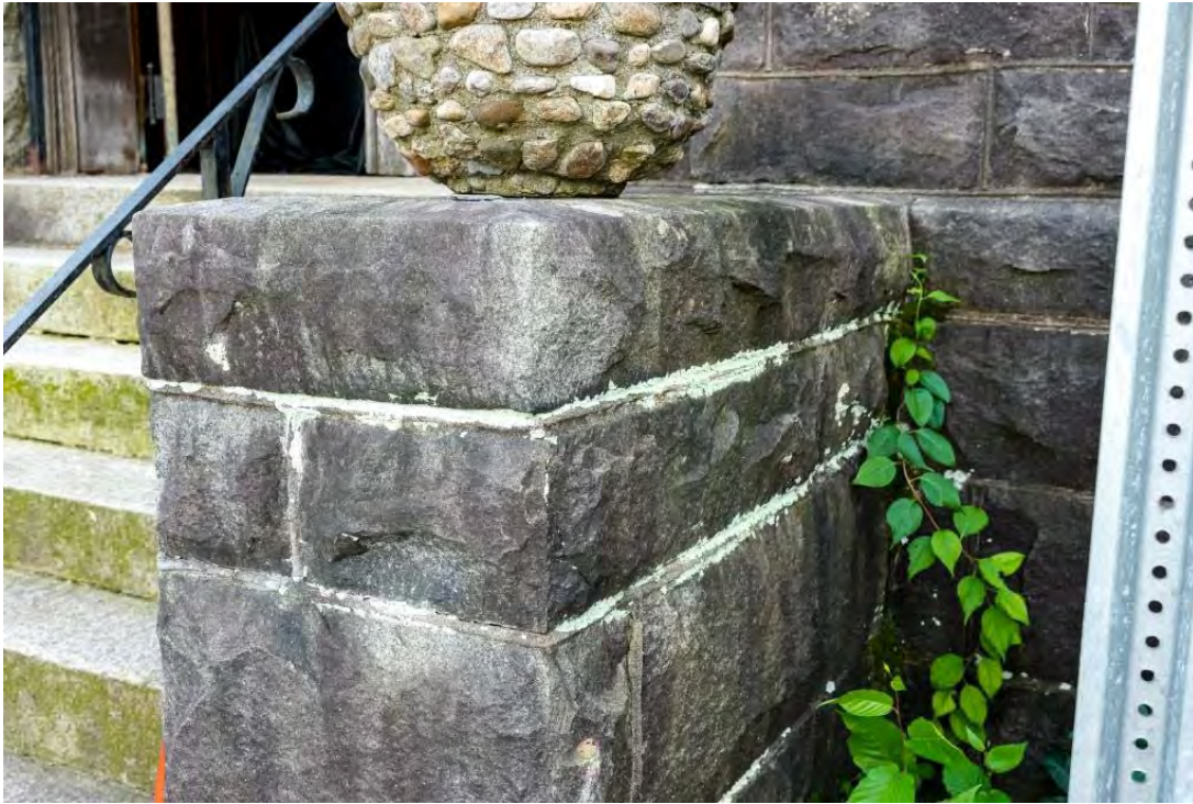
Granite Church – Existing Conditions – Exterior Masonry North, Main Entrance Steps – Staining of in Stone at Sidewalls
