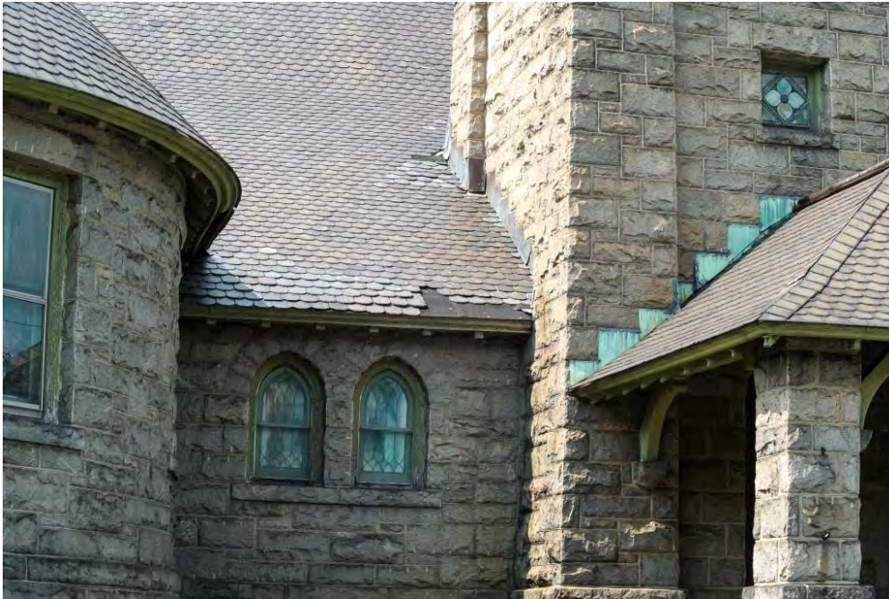
Granite Church – Existing Conditions – Roof and Drainage East Slope of Main Roof - Previous Leaks were an Issue at this Location – Slates Missing – Flashing Damaged Roof/Flashing has been Temporarily Repaired
