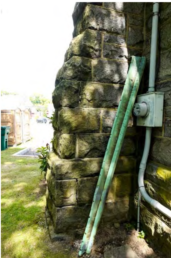
Granite Church – Existing Conditions – Exterior Masonry West Elevation – North Buttress – South Face – Open Joints and Staining
