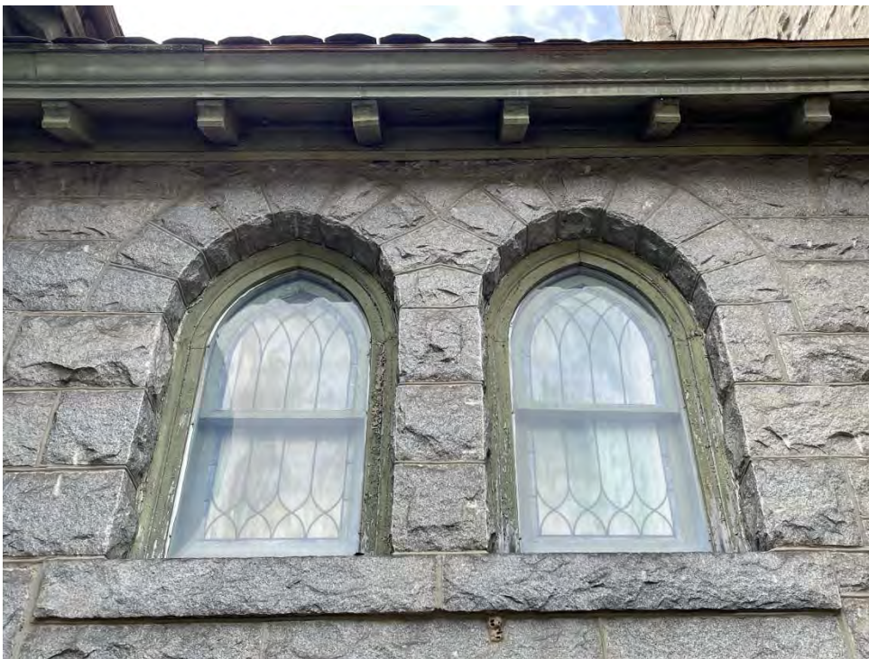
Granite Church – Existing Conditions – Doors and Windows First Floor – Double-Hung Stained-Glass Windows in Stair Hall Exterior View – Frames in Need of Painting
