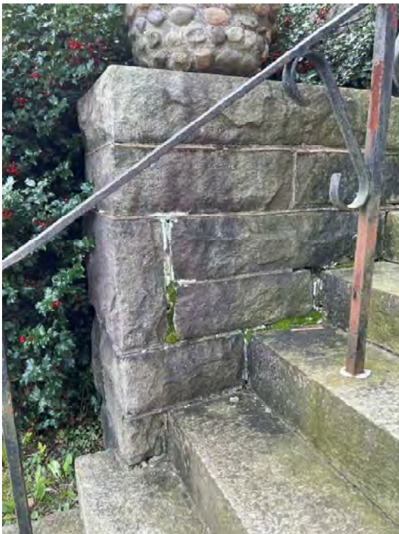
Granite Church – Existing Conditions – Exterior Masonry North, Main Entrance Steps – Open Joints in Stone at Sidewalls
