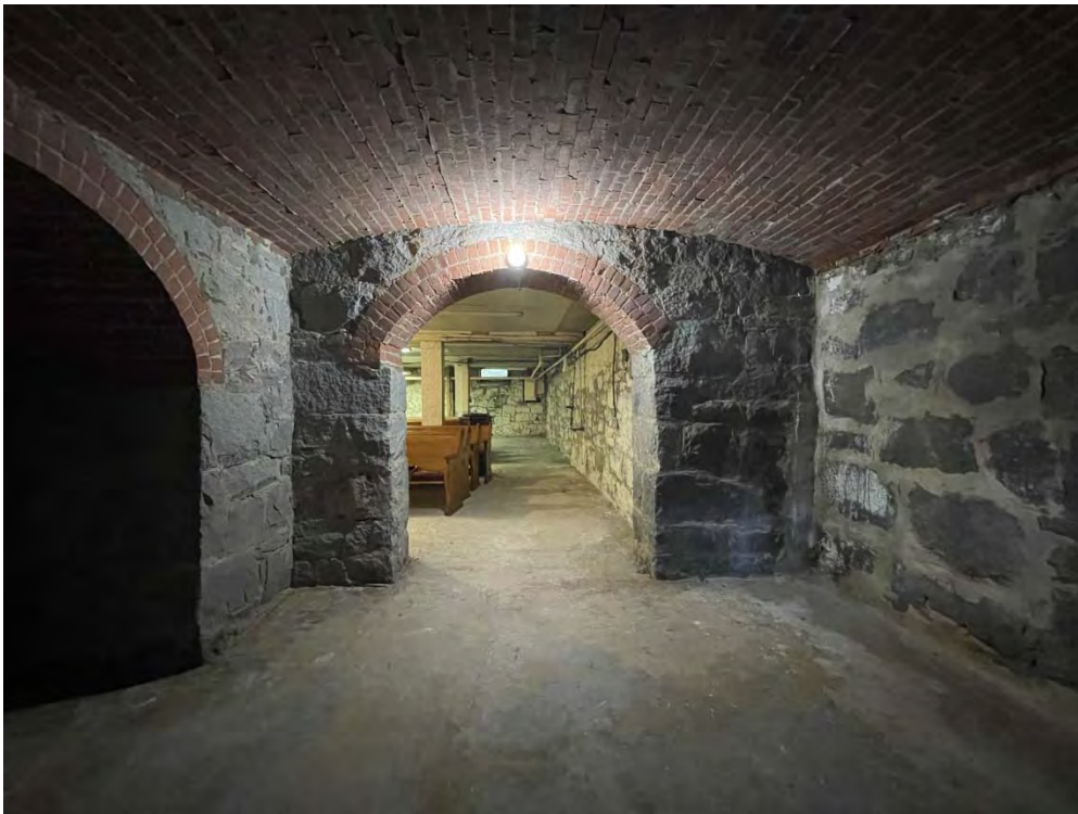
Granite Church – Existing Conditions – Interior Overall Views Basement – Vaulted Room Under Entrance Vestibule Looking West Unfinished Walls, Floor and Ceiling
