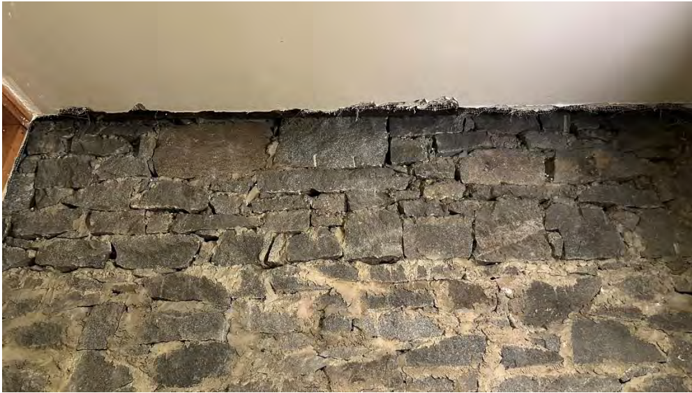
Granite Church – Existing Conditions – Interior Basement – West Room Under Chancel – South Wall Open Joints in Stonework
