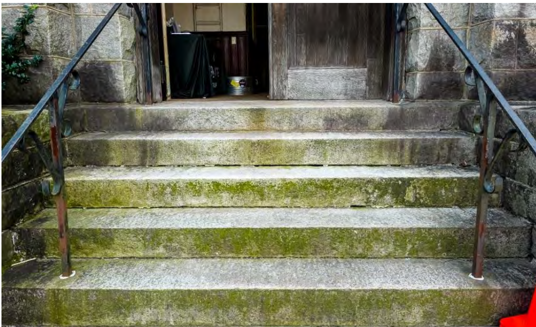
Granite Church – Existing Conditions – Exterior Masonry North, Main Entrance Steps – Open Joints
