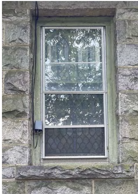
Granite Church – Existing Conditions – Doors and Windows First Floor - Typical Double-Hung Stained-Glass Window on West Wall in Sanctuary Left: Interior View; Right: Exterior View
