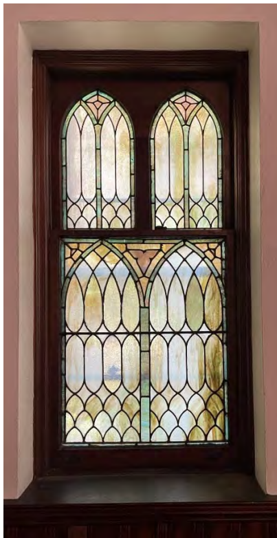
Granite Church – Existing Conditions – Doors and Windows First Floor - Typical Double-Hung Stained-Glass Window on West Wall in Sanctuary Left: Interior View; Right: Exterior View
