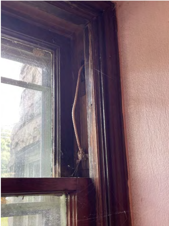
Granite Church – Existing Conditions – Doors and Windows Basement – Double-hung Window in Stair Hall Broken Window Sash Cord
