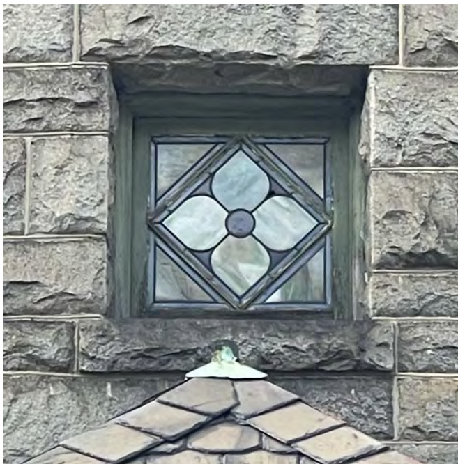
Granite Church – Existing Conditions – Doors and Windows Tower - Typical Fixed Stained-Glass Window Exterior View – Frames in Need of Painting, Generally in Good Condition
