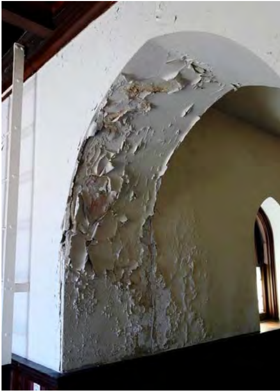
Granite Church – Existing Conditions – Interior Left: Arch in Vestibule; Right: South Wall of Sanctuary Damaged Plaster and Paint due to Previous Roof Leaks
