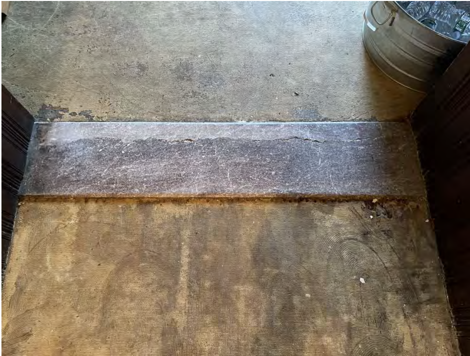
Granite Church – Existing Conditions – Interior First Floor - Stone Threshold Between Entrance Vestibule and Stair Hall Stone is Cracked Longitudinally
