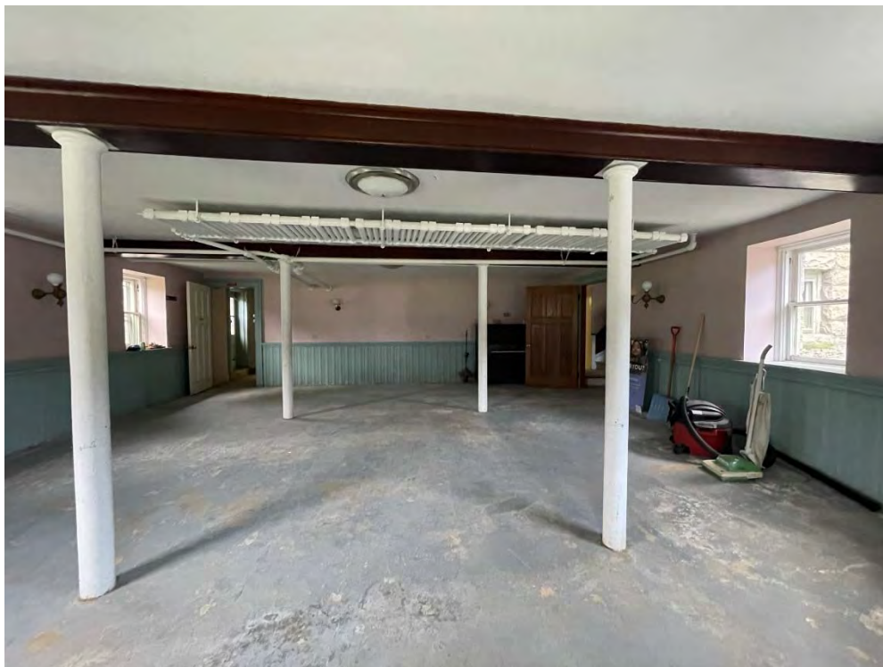
Granite Church – Existing Conditions – Interior Overall Views Basement – East Meeting Room Looking West Finishes Generally in Good Condition; Floor Needs New Surfacing
