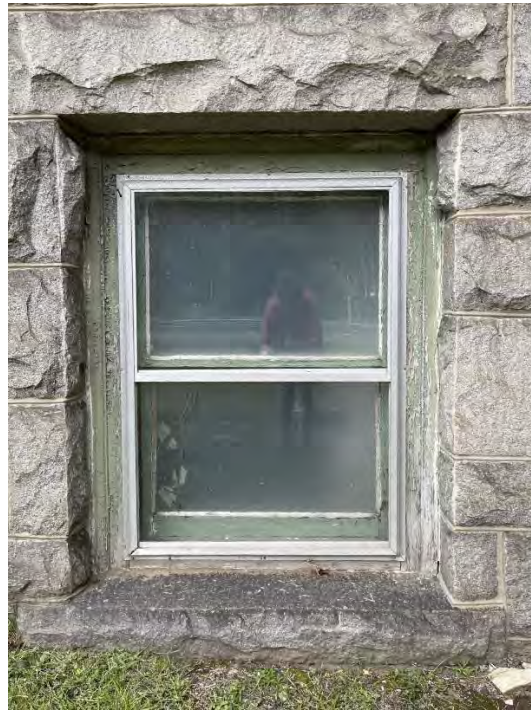
Granite Church – Existing Conditions – Doors and Windows Basement – Typical Double-Hung Window in Women's Toilet Left: Interior View; Right: Exterior View – Wood Frame in Need of Painting, Inappropriate Storms Generally in Good Condition
