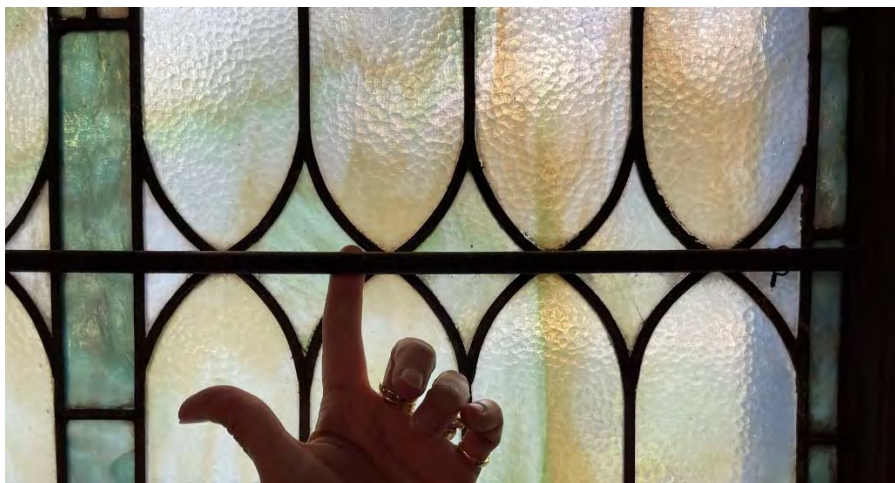
Granite Church – Existing Conditions – Doors and Windows First Floor – Double-Hung Stained-Glass Window on West Wall in Sanctuary – North-most Window Top to Bottom: Bowing of Window, from Left to Right
