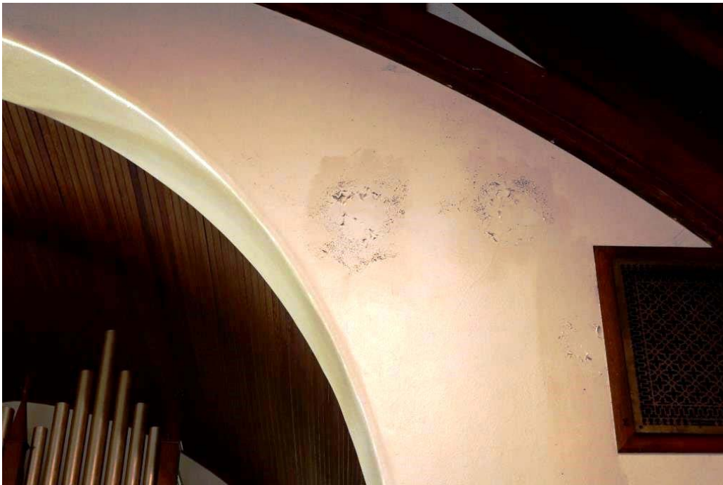
Granite Church – Existing Conditions – Interior South Wall in Sanctuary Damaged Plaster and Paint due to Previous Roof Leaks (Chimney Flashing?)
