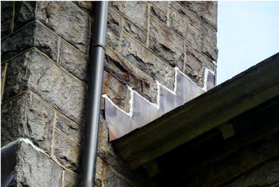
Granite Church – Existing Conditions – Exterior Masonry Chimney at Southwest Corner – South Face – Improper Pointing (Sealant) Staining
