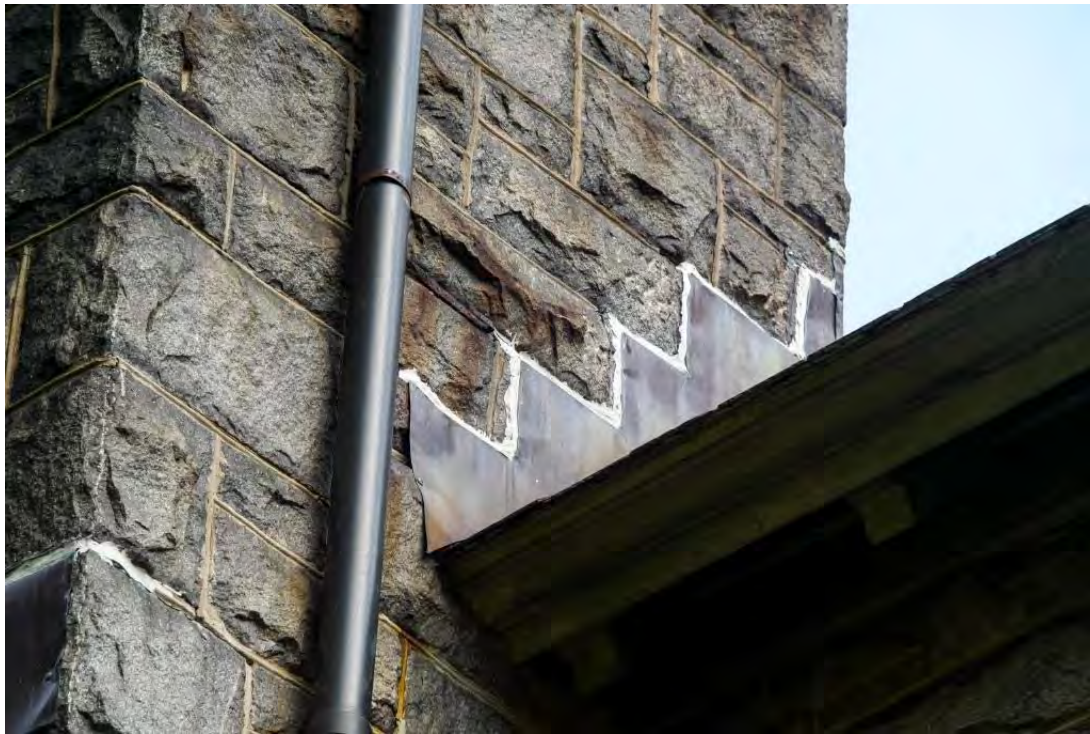
Granite Church – Existing Conditions – Exterior Masonry West Elevation – Chimney at Southwest Corner – South Face – Step Flashing at Chimney to Roof Juncture Appears to be in Good Condition - Improper installation of sealant
