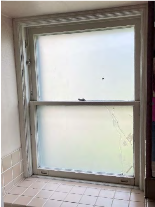
Granite Church – Existing Conditions – Doors and Windows Basement – Typical Double-Hung Window in Women's Toilet Left: Interior View; Right: Exterior View – Wood Frame in Need of Painting, Inappropriate Storms Generally in Good Condition
