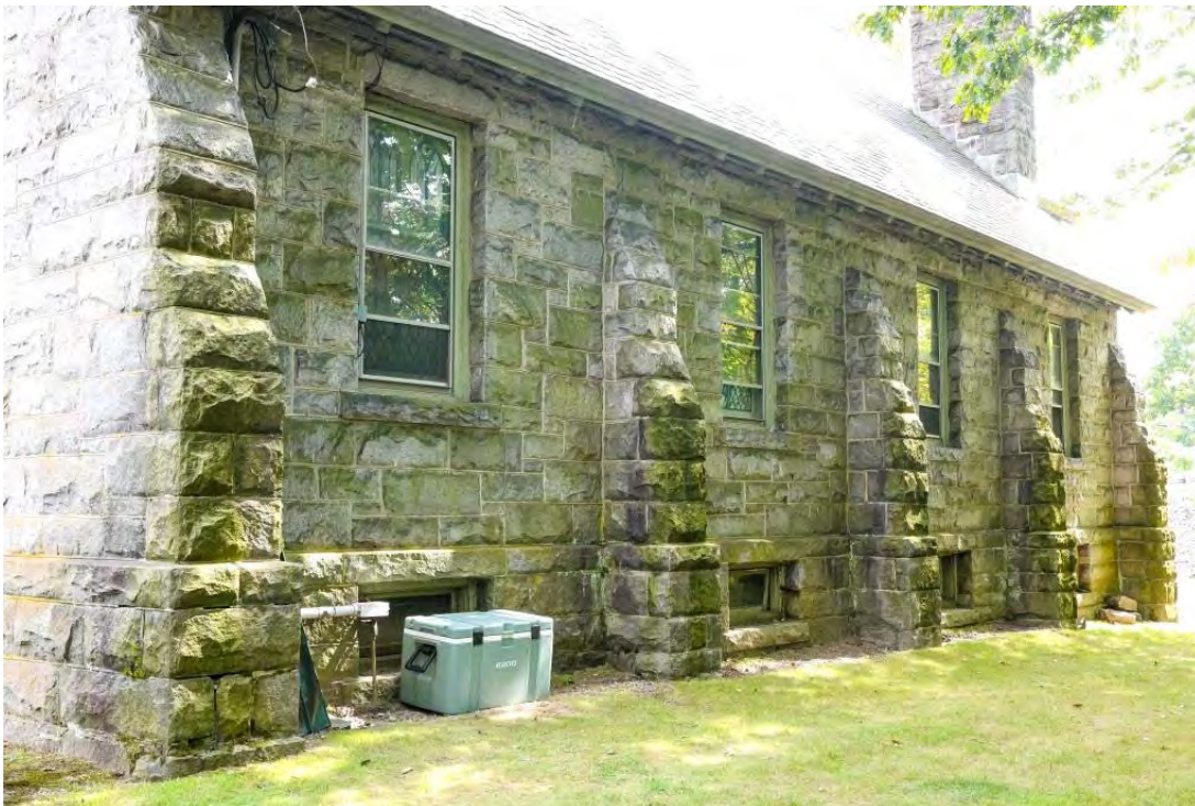
Granite Church – Existing Conditions – Exterior Masonry West Elevation – Overall – Open Joints and Staining
