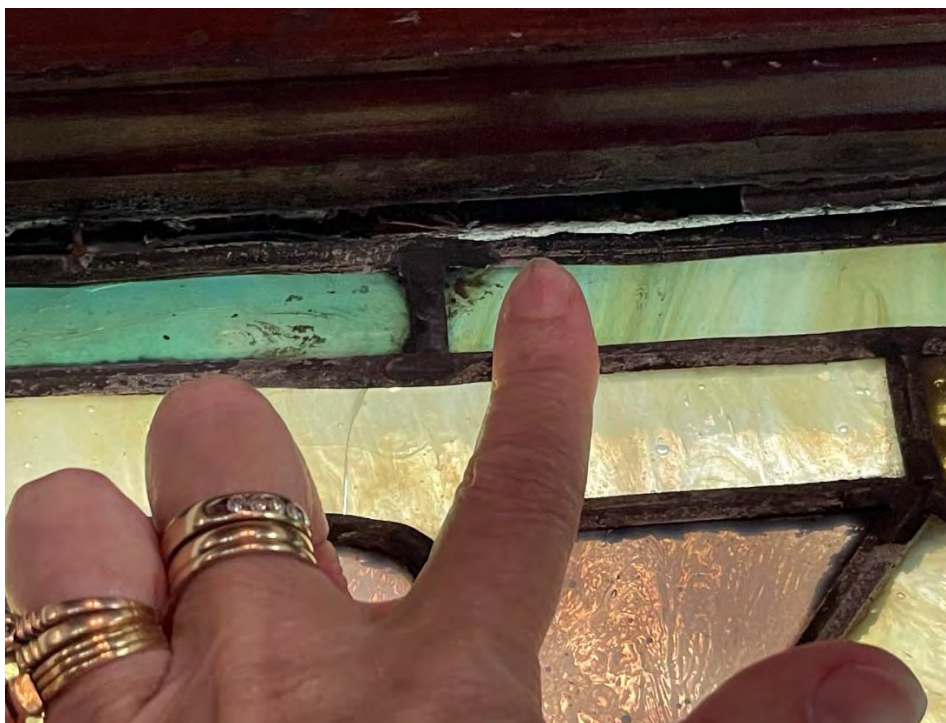
Granite Church – Existing Conditions – Doors and Windows First Floor – Double-Hung Stained-Glass Window on West Wall in Sanctuary – Window Second from South Separation of Window from Frame at top of Bottom Sash
