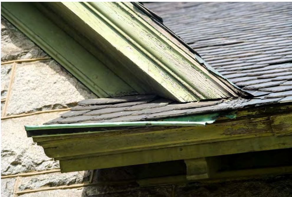
Granite Church – Existing Conditions – Roof and Drainage South Elevation – At Juncture with Semi-Circular East Wing Slates Damaged & Missing – Gutter Missing – Wood Elements Damaged and Lacking Paint
