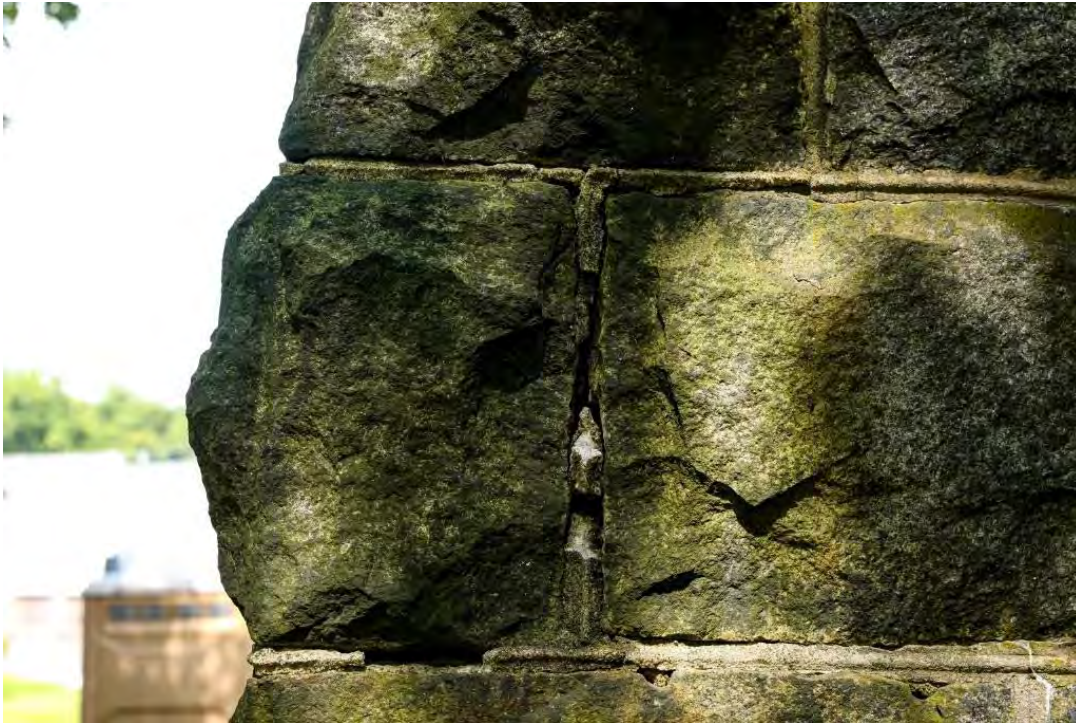
Granite Church – Existing Conditions – Exterior Masonry West Elevation – North Buttress – South Face – Open Joints and Staining
