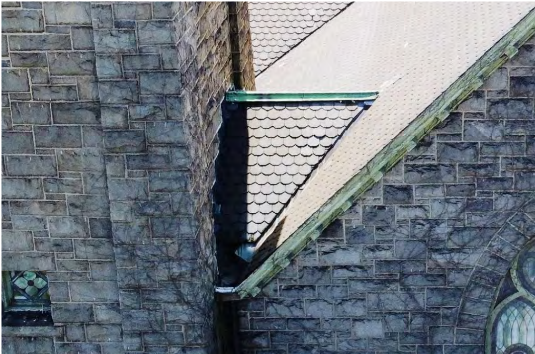
Granite Church – Existing Conditions – Roof and Drainage Cricket on North Side of Tower – Previous Leaks were an Issue at this Location Roof/Flashing has been Temporarily Repaired
