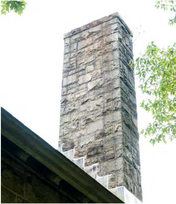
Granite Church – Existing Conditions – Exterior Masonry West Elevation – Chimney at Southwest Corner – North and West Faces - Staining
