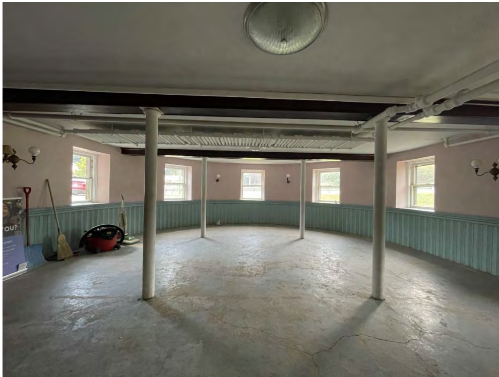
Granite Church – Existing Conditions – Interior Overall Views Basement – East Meeting Room Looking East Finishes Generally in Good Condition; Floor Needs New Surfacing
