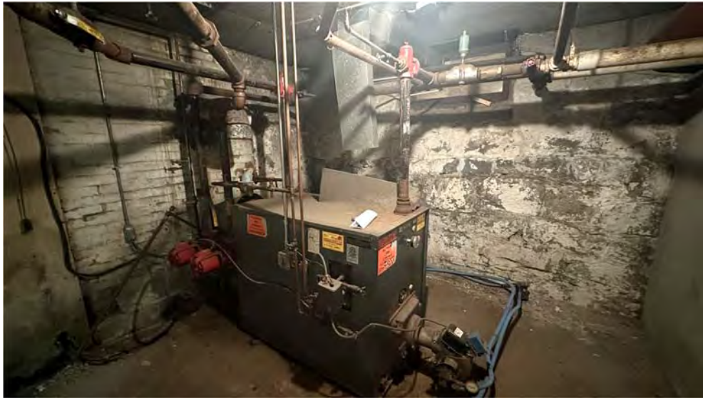
Granite Church – Existing Conditions – MEP Basement – Existing Gas Fired Boiler Boiler is Disconnected and Fuel Tanks Have Been Removed
