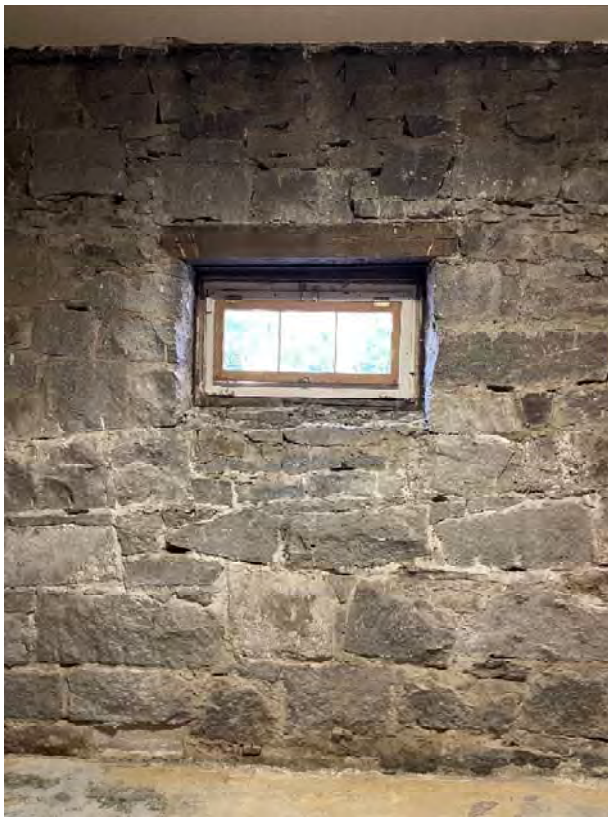
Granite Church – Existing Conditions – Interior Basement – West Room Under Chancel – West Wall Open Joints in Stonework
