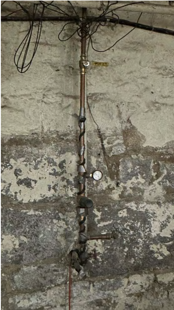
Granite Church – Existing Conditions – MEP Basement – Main Water Service Entrance Water supply currently turned off
