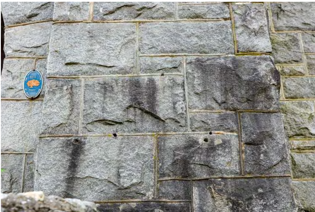
Granite Church – Existing Conditions – Exterior Masonry North Wall West of Main Entrance – Holes in Stonework at Removed Plaque
