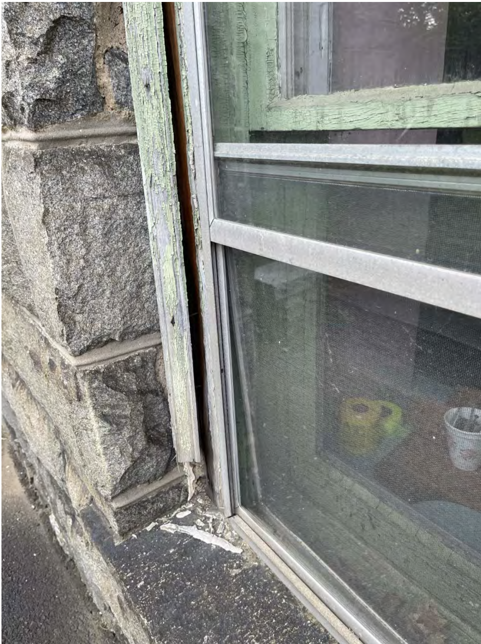
Granite Church – Existing Conditions – Doors and Windows Basement – Double-Hung Window in East Meeting Room - West-most Window on South Wall Damaged Wood Trim, Windows in Need of Paint, Damaged Storm Window
