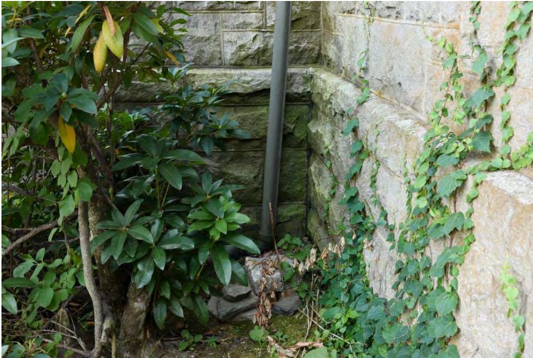
Granite Church – Existing Conditions – Exterior Masonry North Elevation – Northwest Inside Corner beside Tower Vegetation on Stonework – Drainage Issues at Base of Leader – Staining at Base of Wall
