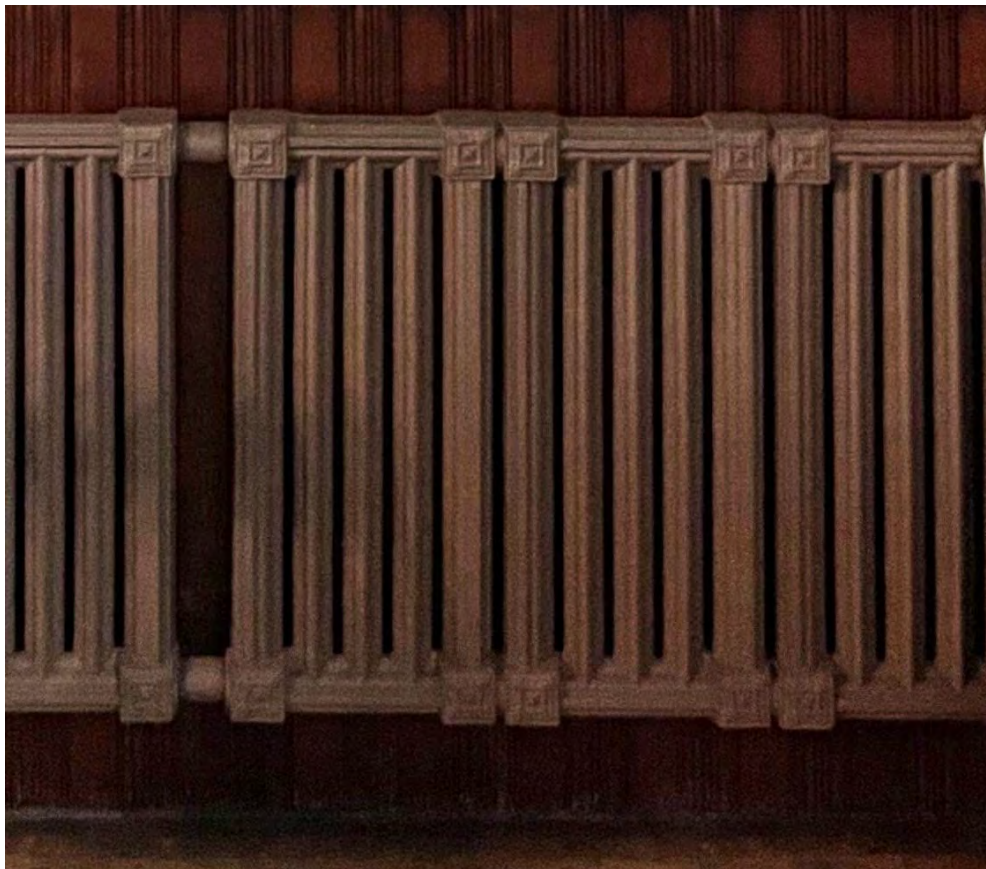
Granite Church – Existing Conditions – MEP First Floor – Sanctuary – Typical Existing Hot Water Radiator
