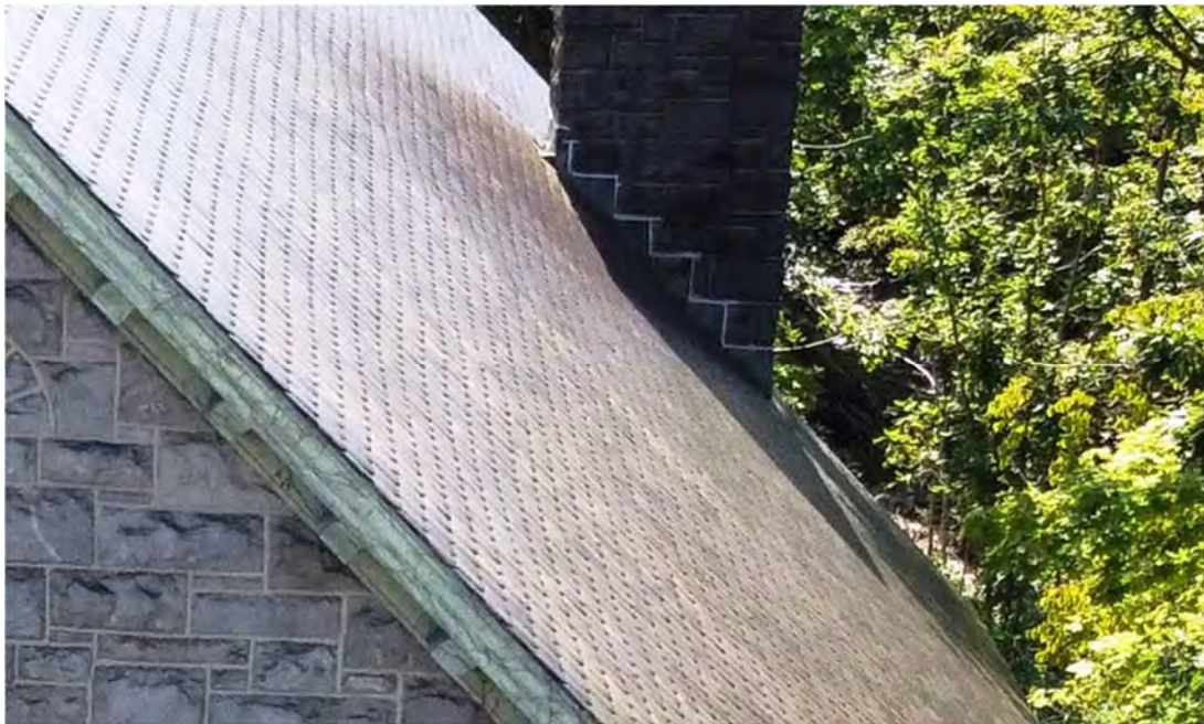
Granite Church – Existing Conditions – Exterior Masonry Chimney at Southwest Corner – North Face – Step Flashing at Chimney to Roof Juncture Appears to be in Good Condition; No Cricket at East Face of Chimney
