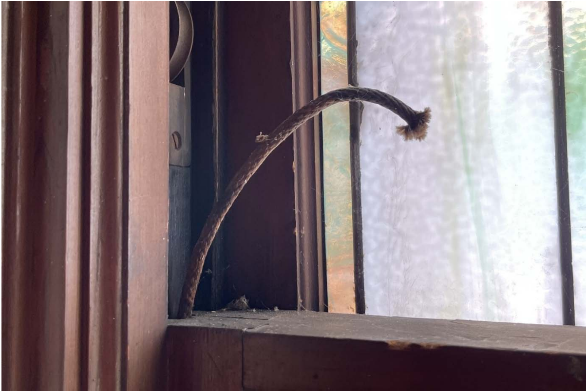
Granite Church – Existing Conditions – Doors and Windows First Floor – Double-Hung Stained-Glass Windows in Stair Hall Broken Window Cord
