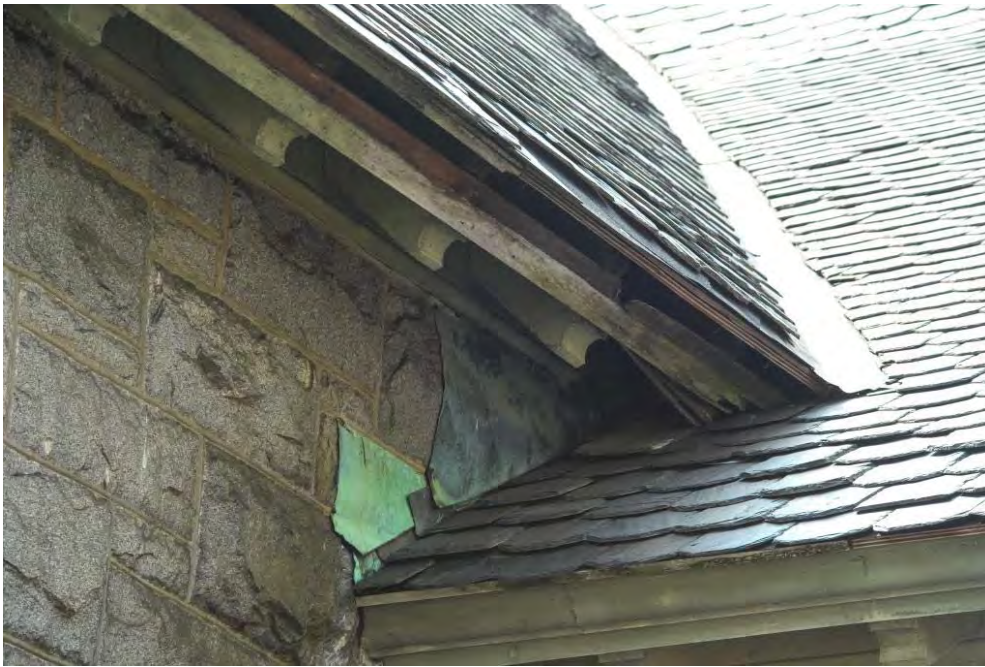
Granite Church – Existing Conditions – Roof and Drainage East Slope of Main Roof – At Juncture with North Wall of Semi-Circular East Wing Slates Missing – Flashing Damaged – Gutter Missing - Wood Elements Damaged and Lacking Paint Roof/Flashing has been Temporarily Repaired
