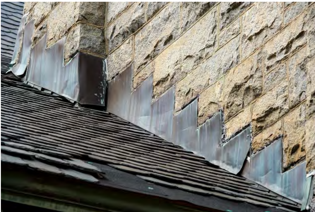
Granite Church – Existing Conditions – Roof and Drainage East Slope of Main Roof – Detail - Previous Leaks were an Issue at this Location - Slates Missing – Flashing Damaged Roof/Flashing has been Temporarily Repaired
