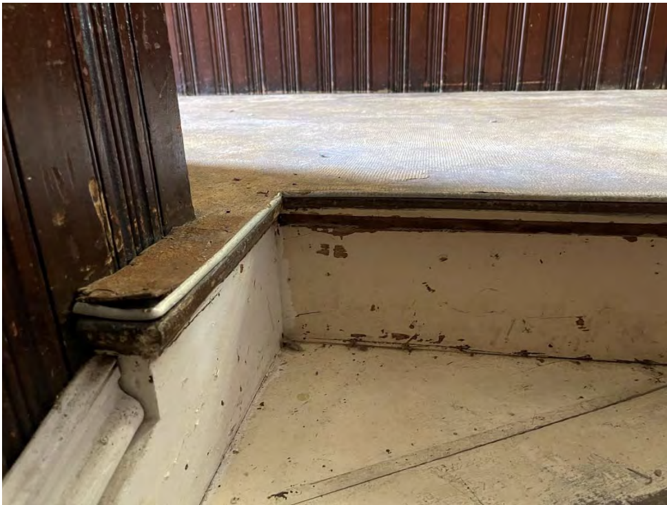
Granite Church – Existing Conditions – Interior First Floor - Stair Hall Original Wood Floor covered by Fiberboard Subfloor; Vinyl Tile has been Removed
