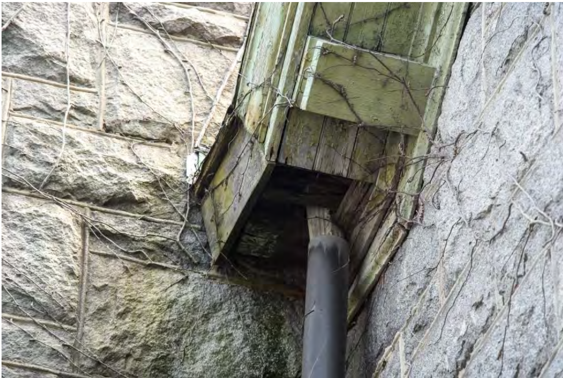
Granite Church – Existing Conditions – Roof and Drainage Drain and Downspout from Main Roof at Intersection with North Side of Tower – Wood Fascia and Soffit Missing -
