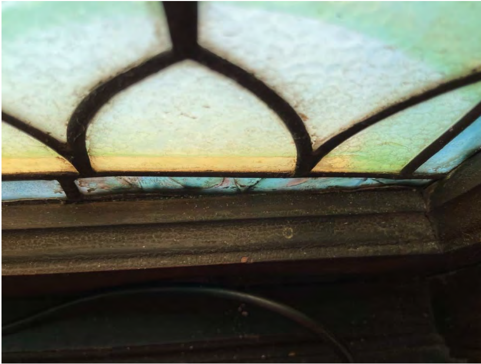
Granite Church – Existing Conditions – Doors and Windows First Floor – Double-Hung Stained-Glass Window in East Meeting Room – East-most Window Deflection of Lead Comes and Glass at Base of Window
