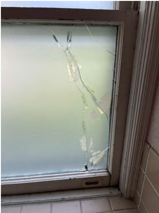
Granite Church – Existing Conditions – Doors and Windows Basement – Double-Hung Window in Women's Toilet Cracked Glass
