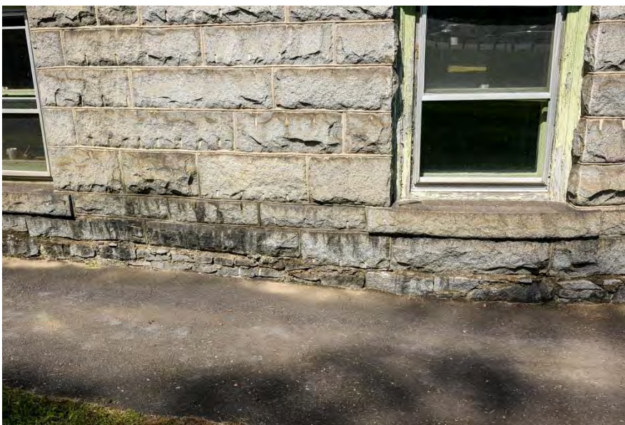
Granite Church – Existing Conditions – Exterior Masonry East Elevation – East Wall of Chancel – Staining at Base of Wall
