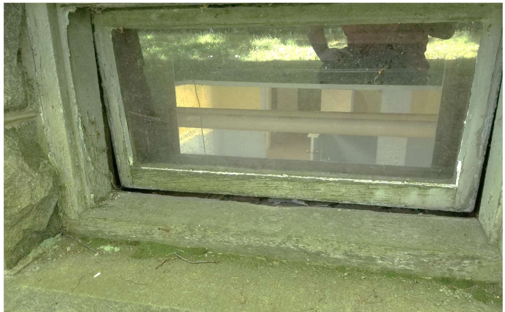
Photo 11: Peeling paint and beginnings of rot in basement window.
