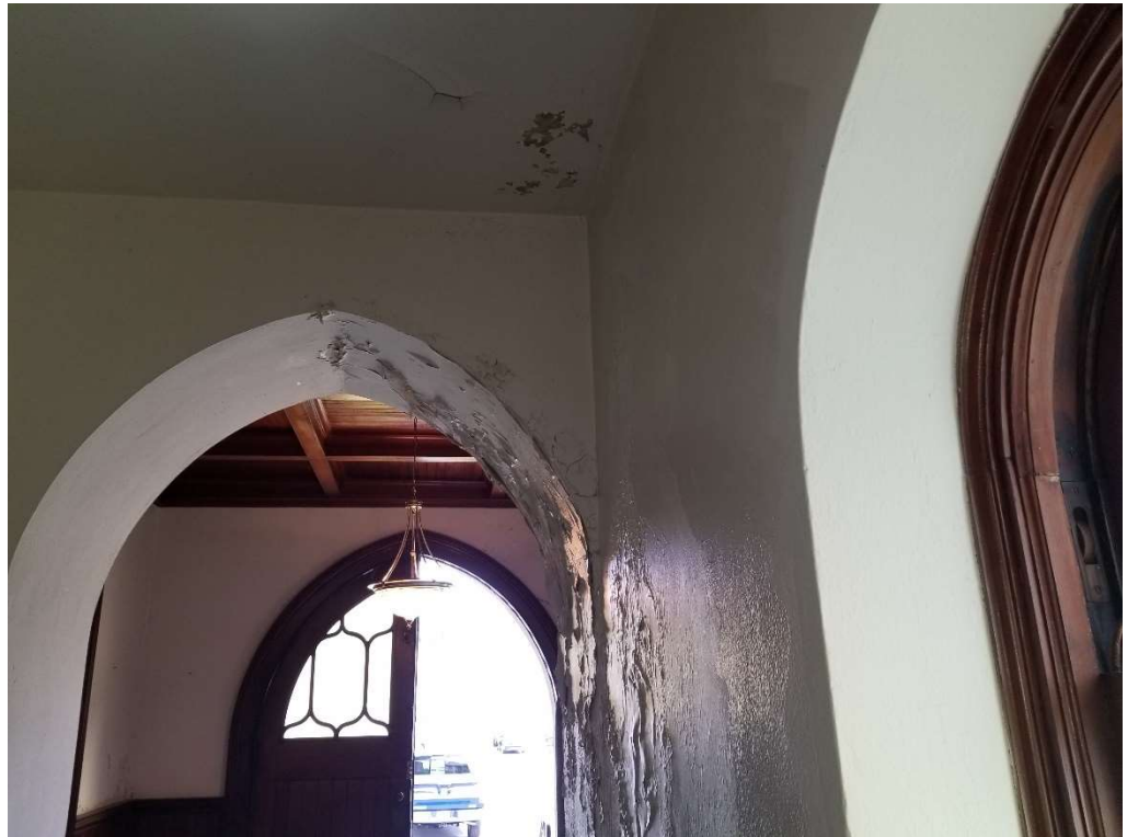
Photo 25: Heavy water damage to plaster walls at archway.
