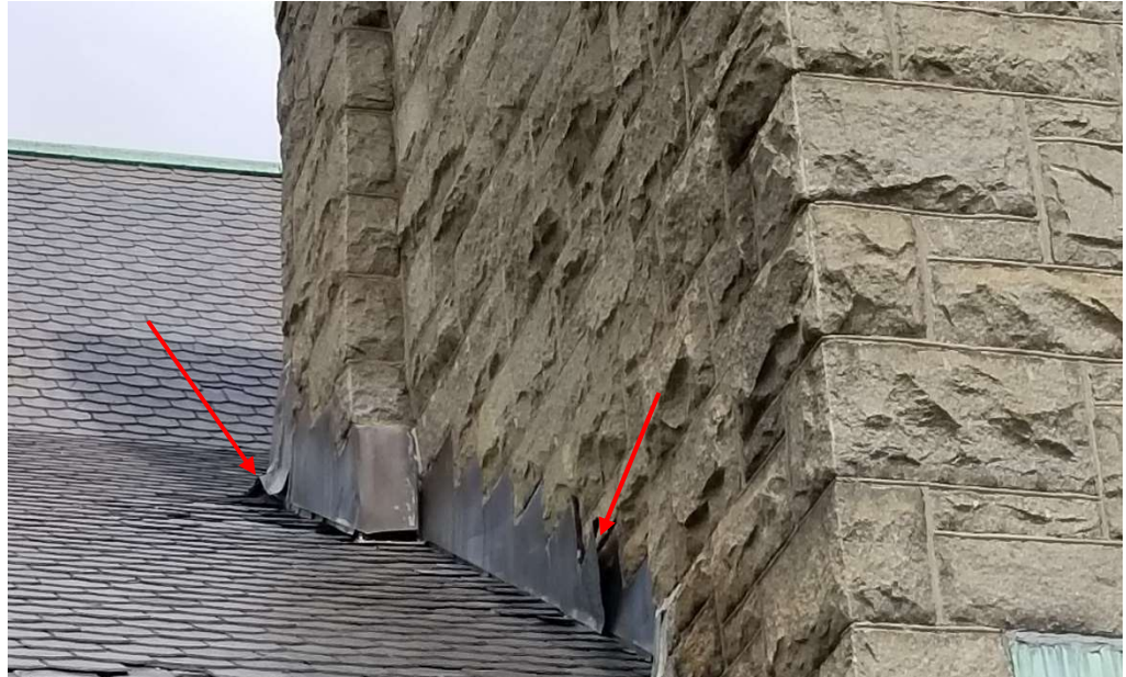
Photo 23: Damaged sawtooth counter flashing.
