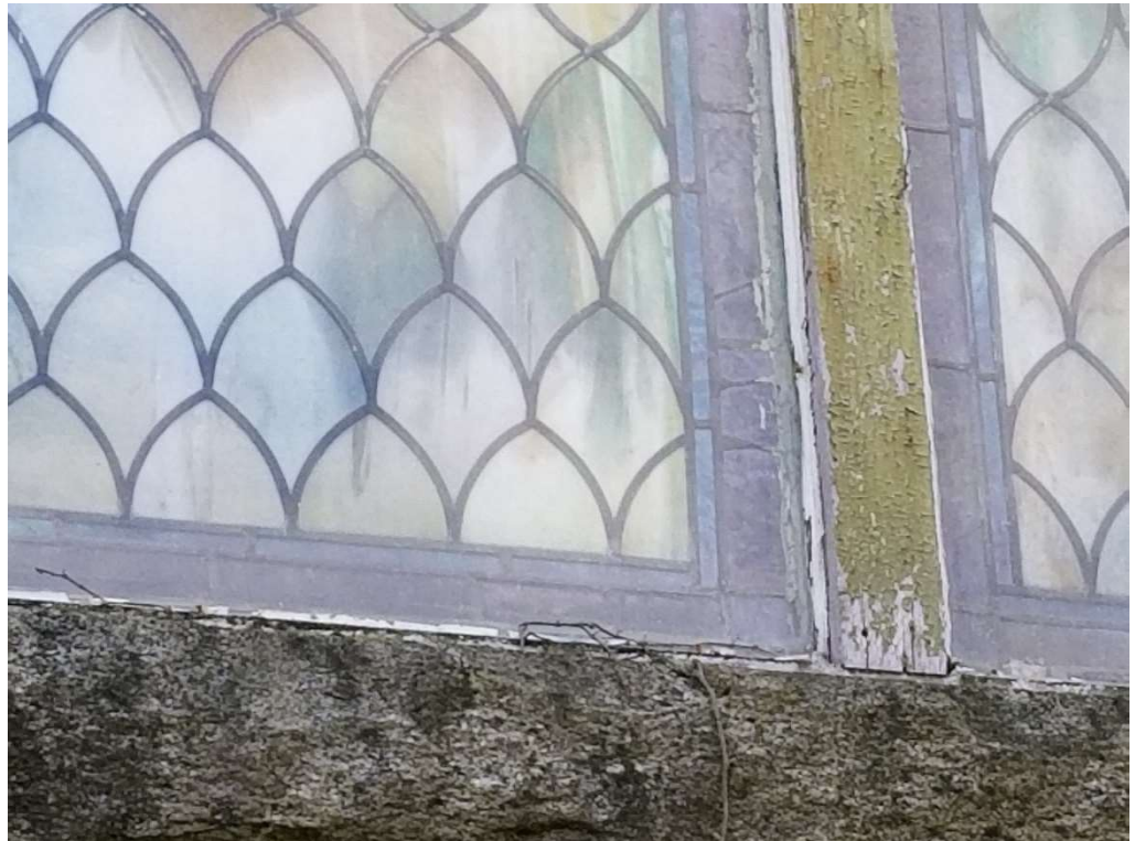
Photo 16: Stained glass window showing peeling paint, wood rot and failed glazing sealant.
