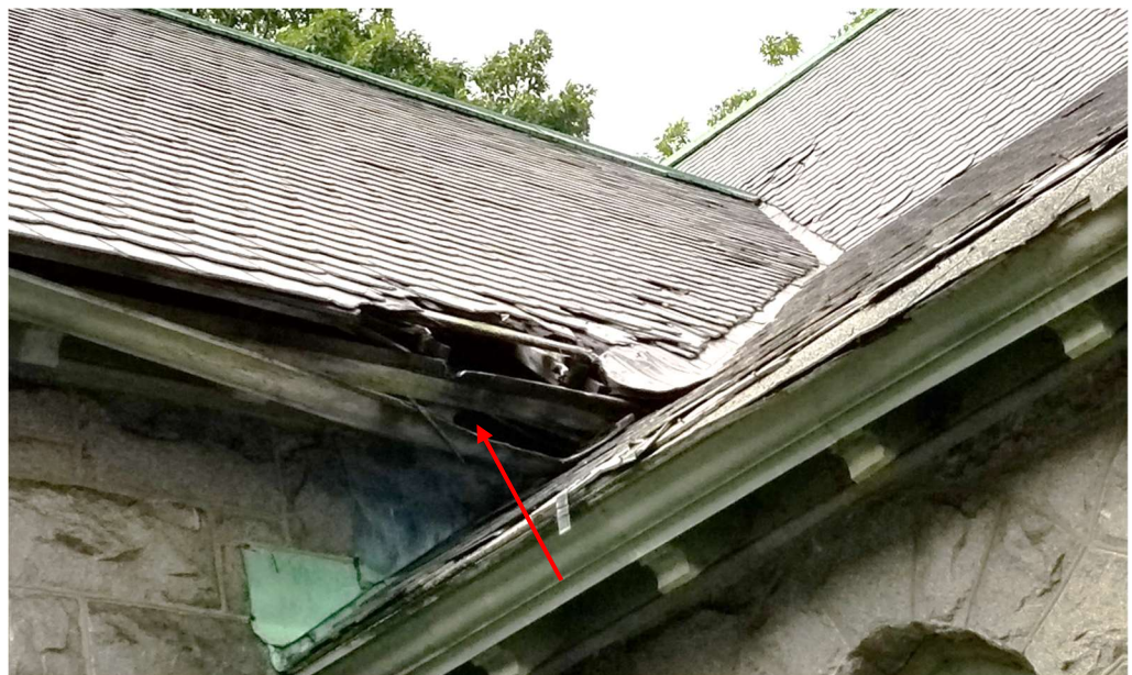
Photo 21: Damage to roof decking and eave molding. Also note, no gutters at the eaves.
