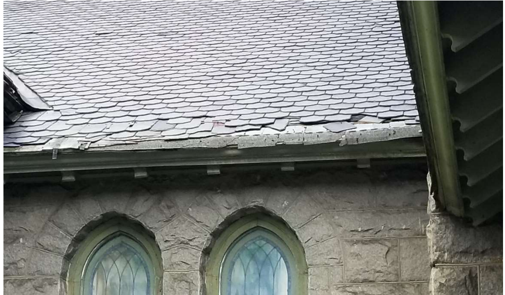
Photo 20: Missing slate at eave replaced with asphalt shingles.
