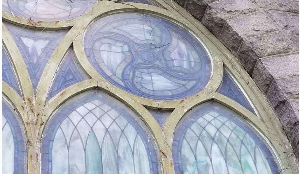
Photo 14: Rust stains, peeling paint and the beginning of wood rot in window.
