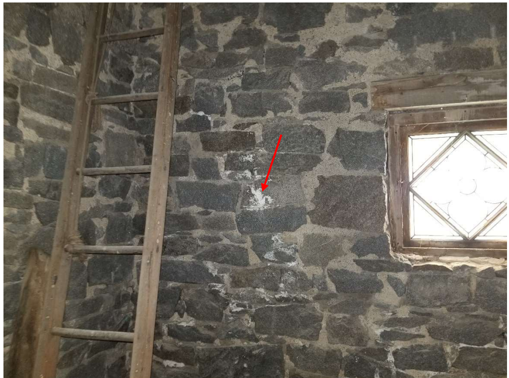
Photo 17: Efflorescence in bell tower.
