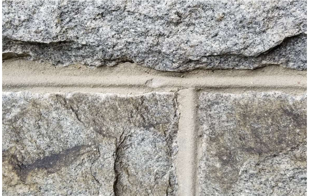
Photo 6: Beaded mortar joints in good condition.
