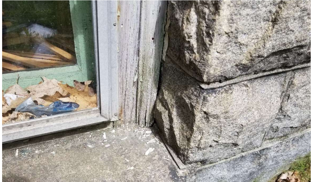
Photo 9: Peeling paint and the beginnings of dry rot in wood window.
