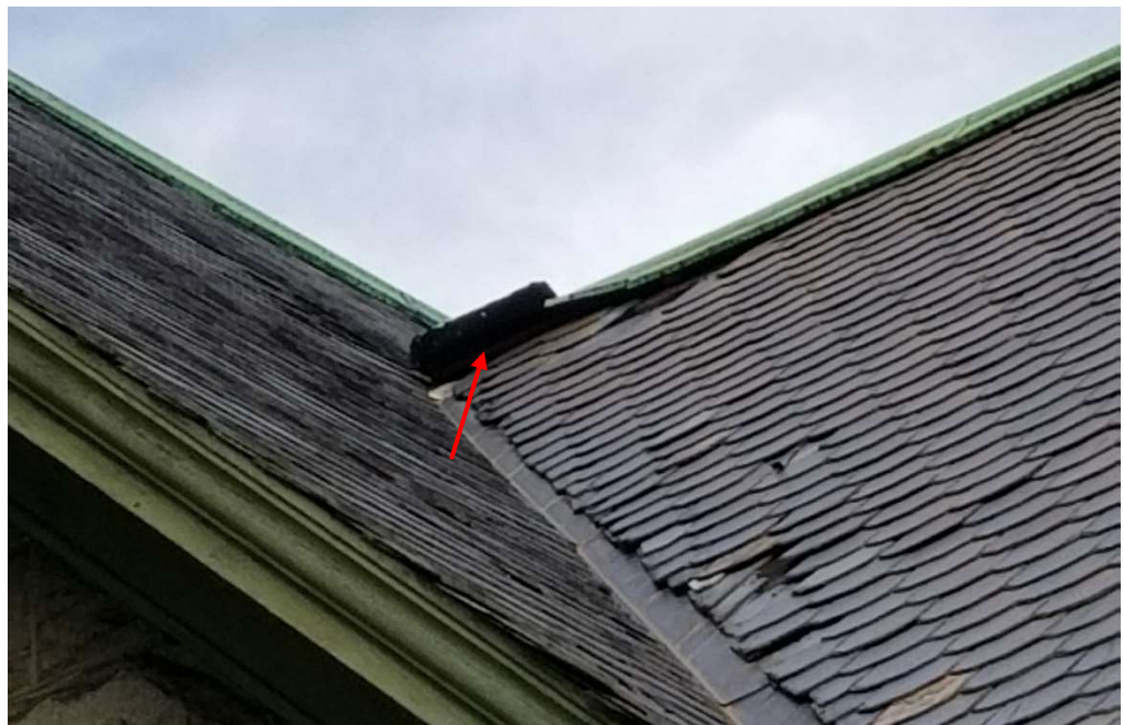
Photo 24: Damaged ridge flashing.
