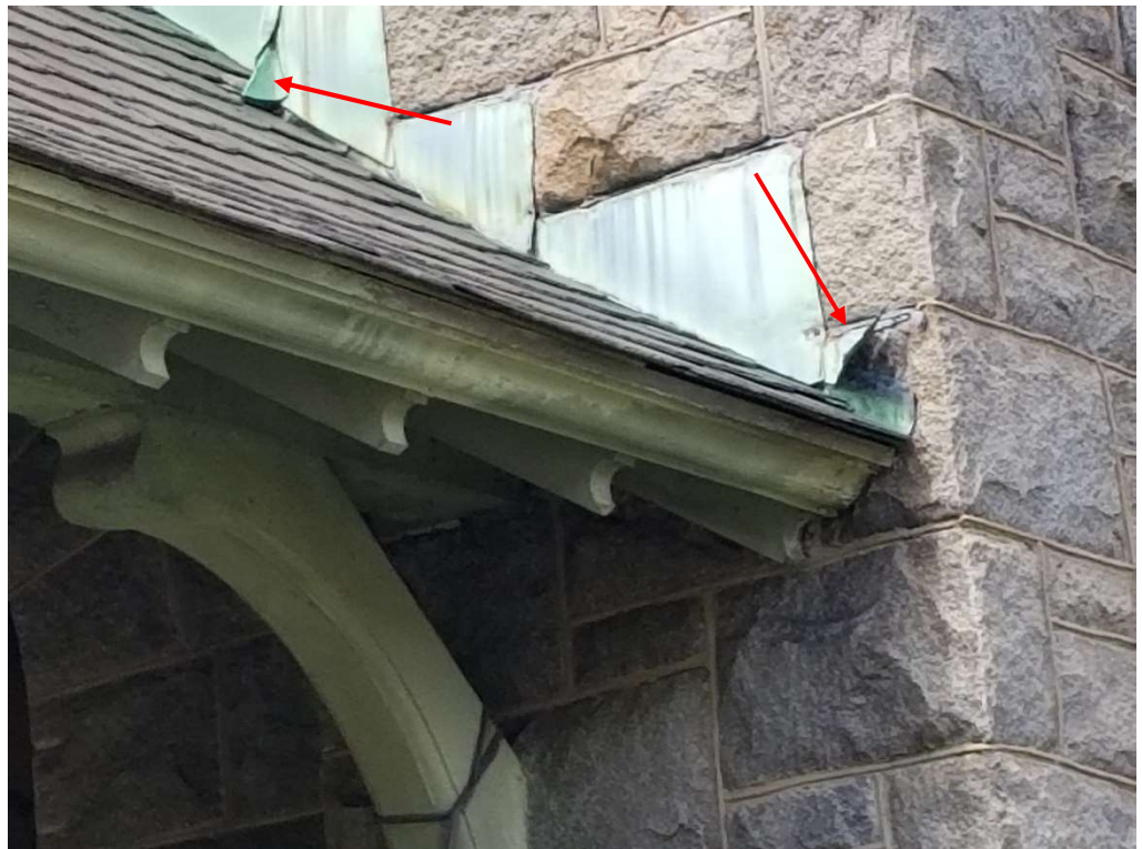
Photo 22: Damaged copper step flashing.
