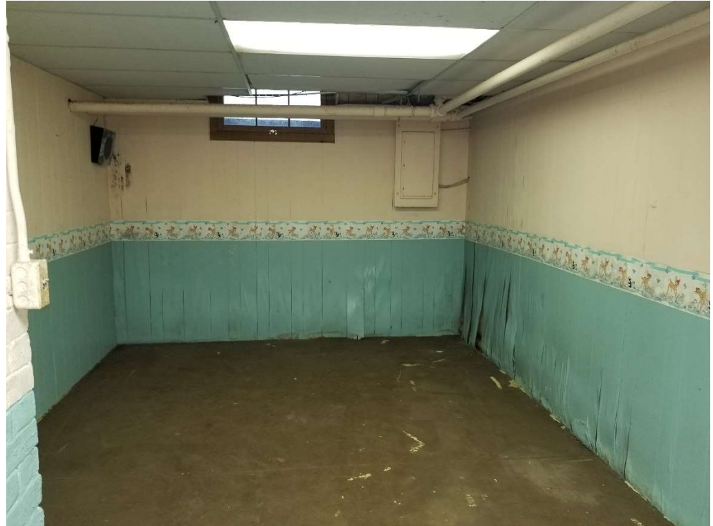
Photo 26: Water damage to interior finishes in basement.
