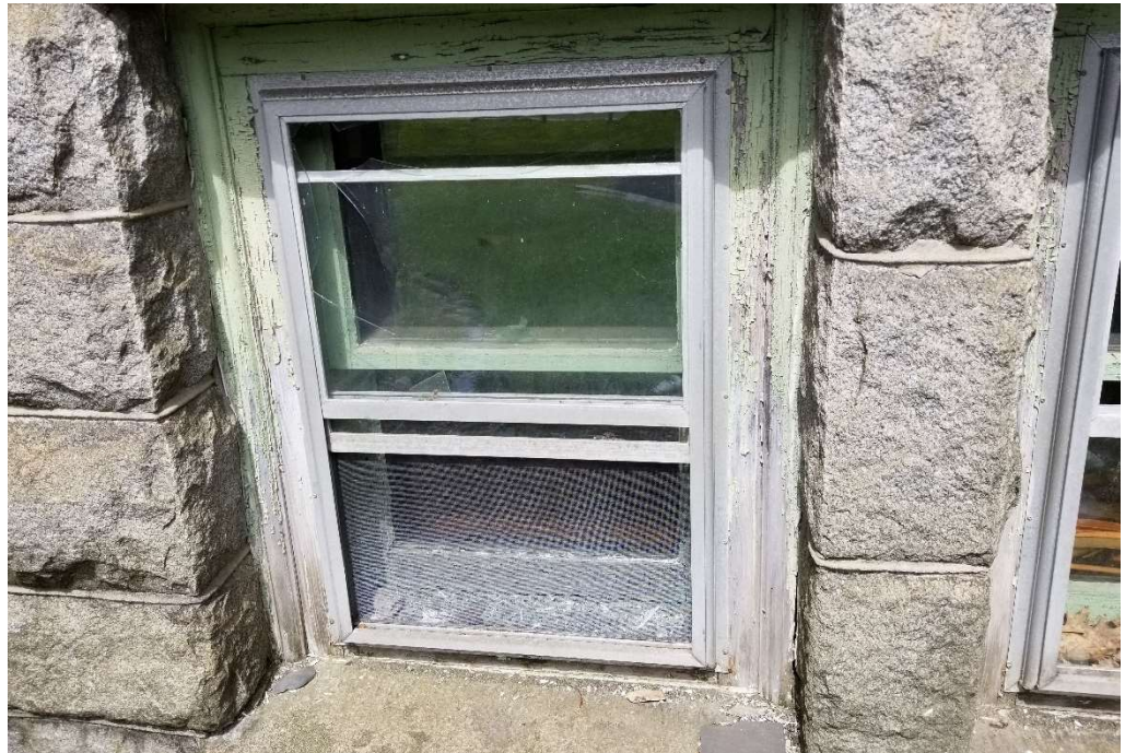
Photo 12: Peeling paint on window frame and broken storm window.
