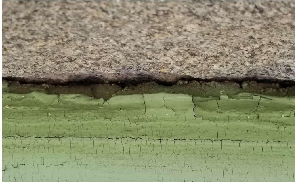
Photo 10: Dried and cracked sealant at perimeter of window.
