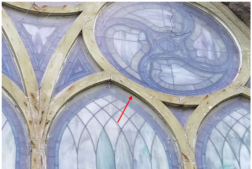
Photo 15: Dried and cracked glazing sealant.
