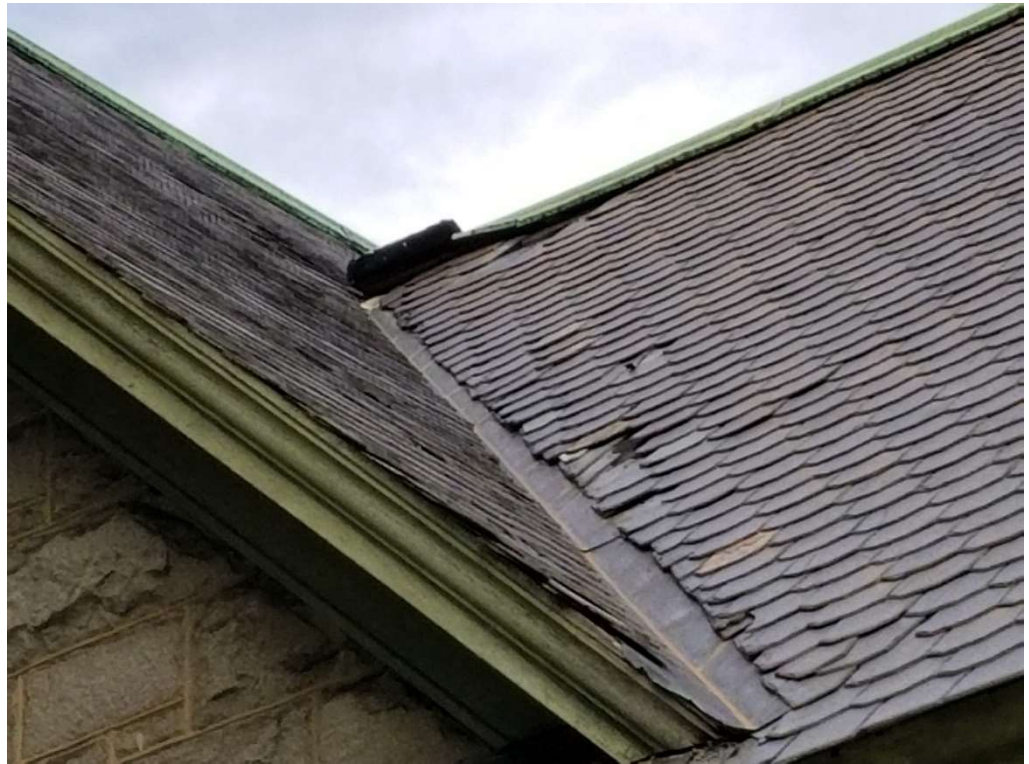
Photo 19: Broken, missing and loose slate.
