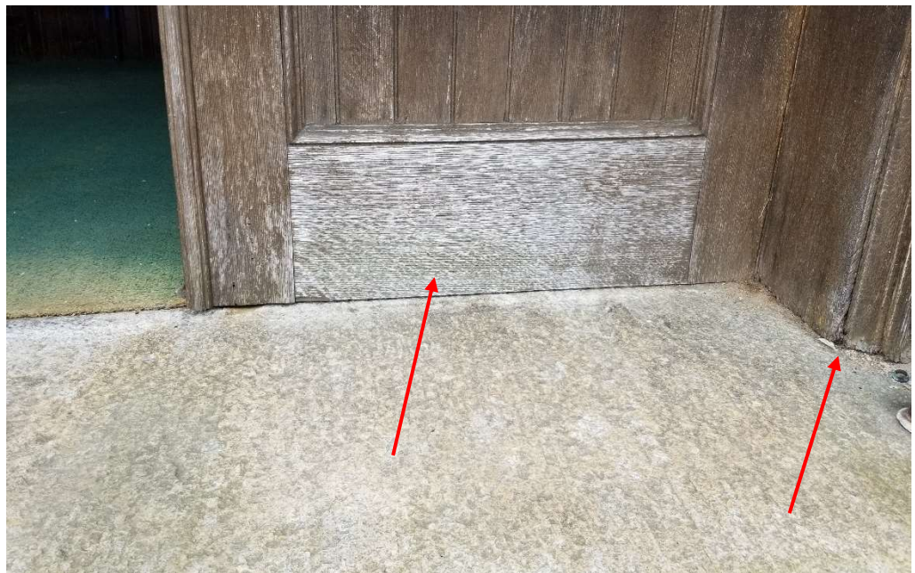
Photo 4: Water damage and rot at the base of wood door.
