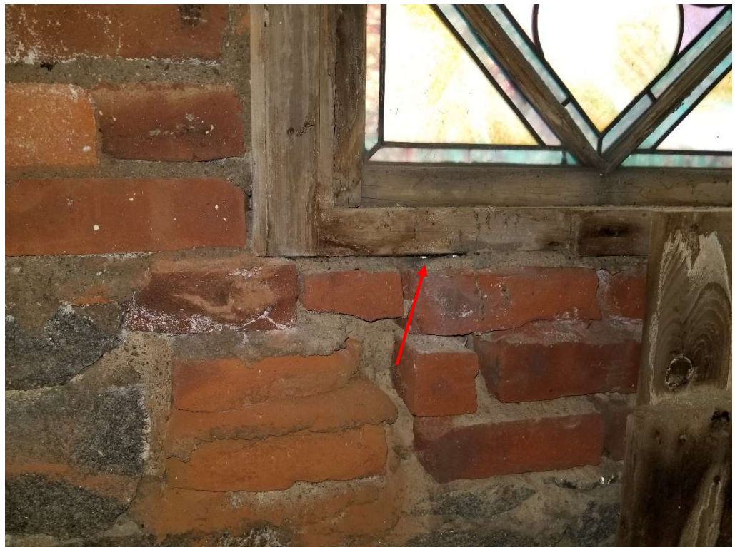
Photo 18: Daylight at window perimeter.
