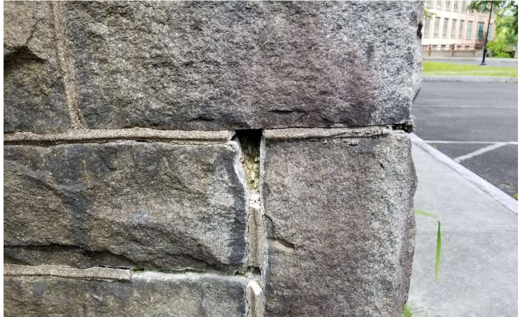
Photo 3: Mortar erosion at parapets.
