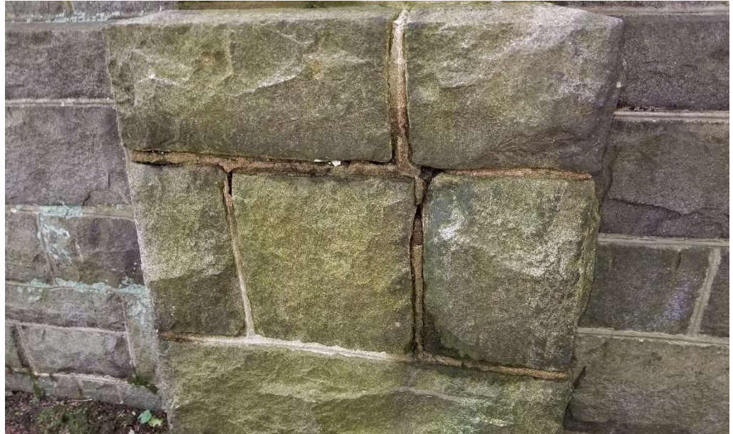
Photo 8: Eroded mortar joints.
